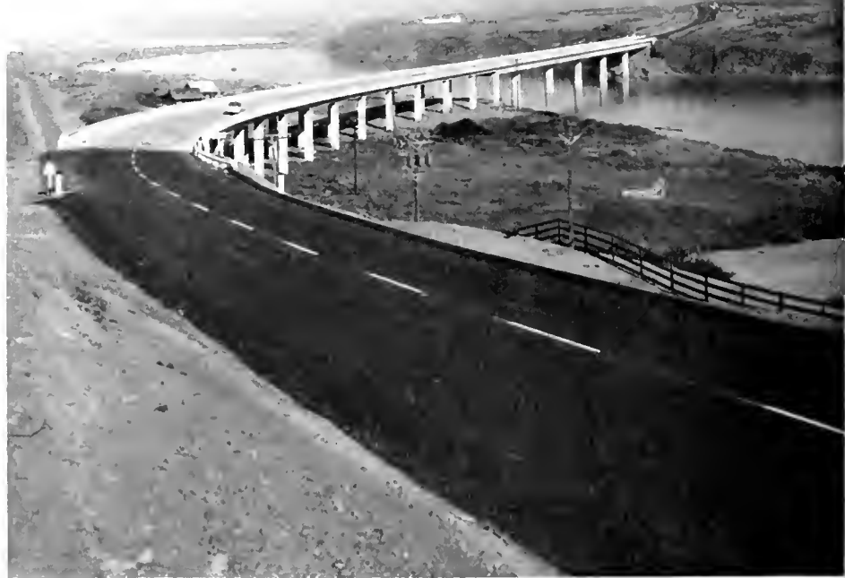
New Ten Mile River Bridge in Mendocino County
